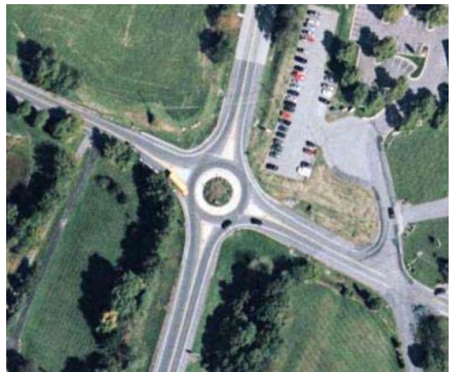
Single Lane Roundabout in Lisbon, MD
