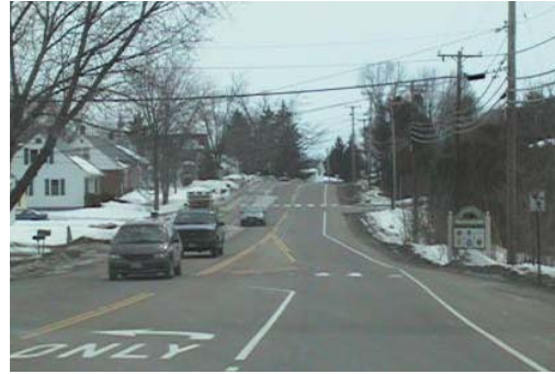
Wide Paved Shoulder
